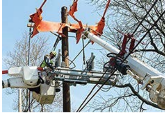
Figure 2-9. Workers Rebuilding a Transmission Line (Fischbach, 2014)
