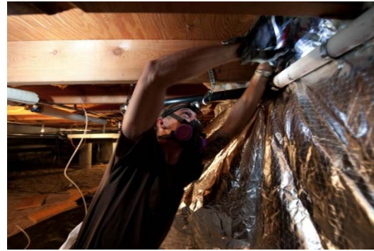
Figure 2-15. Adding Insulation in an Existing Home (U.S. DOE, 2015a)
